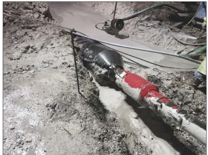
Figure 7. Leading Head of Fusible Polyvinyl Chloride Pipe
