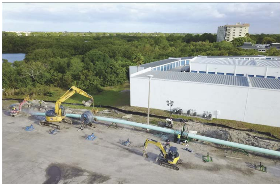
Figure 4. Fusible Polyvinyl Chloride Installation and Fusing Operations
